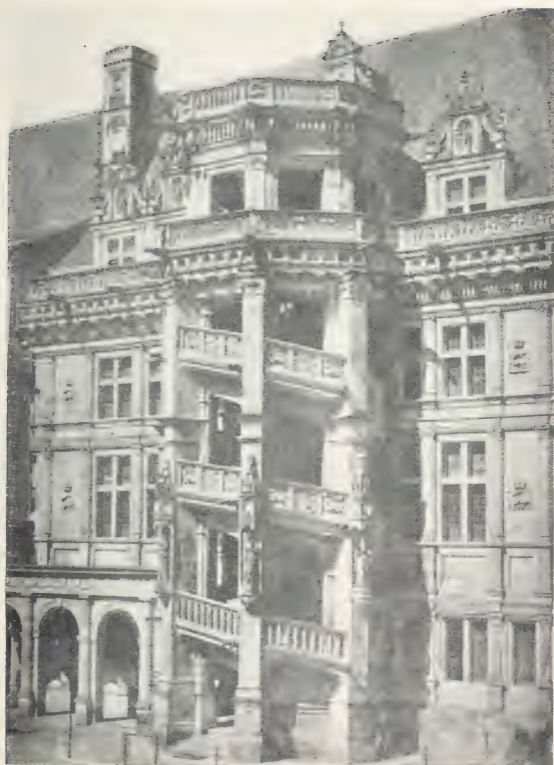
BLOIS: STAIRCASE OF FRANCIS I
